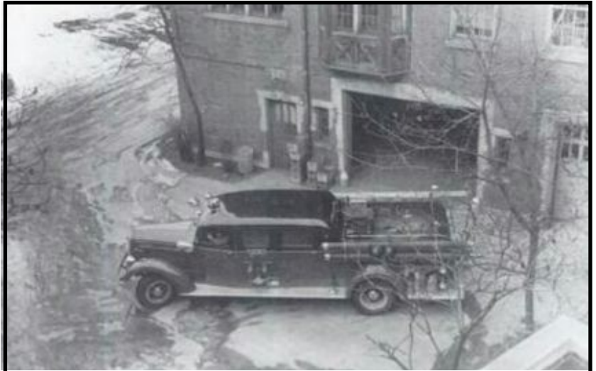
One of the shortcomings of the Civic Center was the fire department being placed in the narrow back alley. It required the engine to make three point turns to enter and exit the garage—not great in an emergency.
